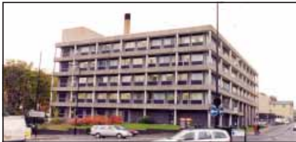
• Ridley Building, Queen Victoria Road
